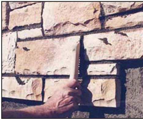
5. Use a wire brush to clear away chunks of excess mortar in the joint and on the surface of the stone. Do not allow mortar to dry on surface.
