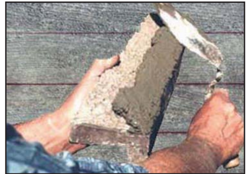
Applying mortar to stone
