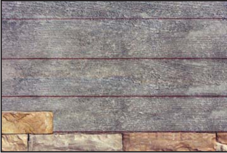
Applying First course of stone
