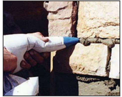
3. Fill the grout joints. Make a fist and push into the bag to force mortar into the joints.
