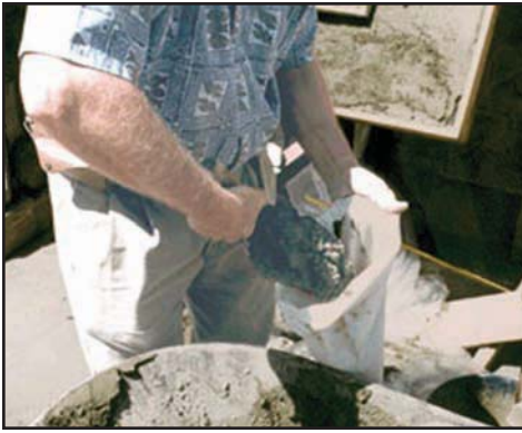
1. Fill grout bag using a trowel.
