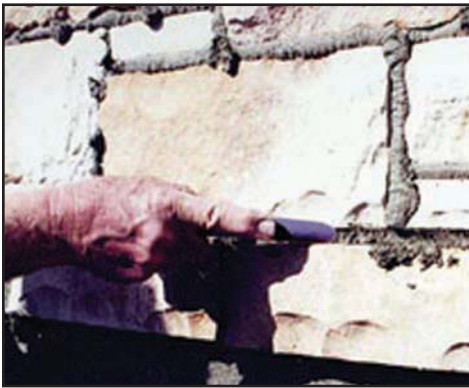
4. Using the back of a wire brush, stick or something similar, press the mortar into the joints as the mortar is beginning to set and before it gets too hard. When this process is done too soon the mortar can smear on the face of the stone or give the grout a slick look.
